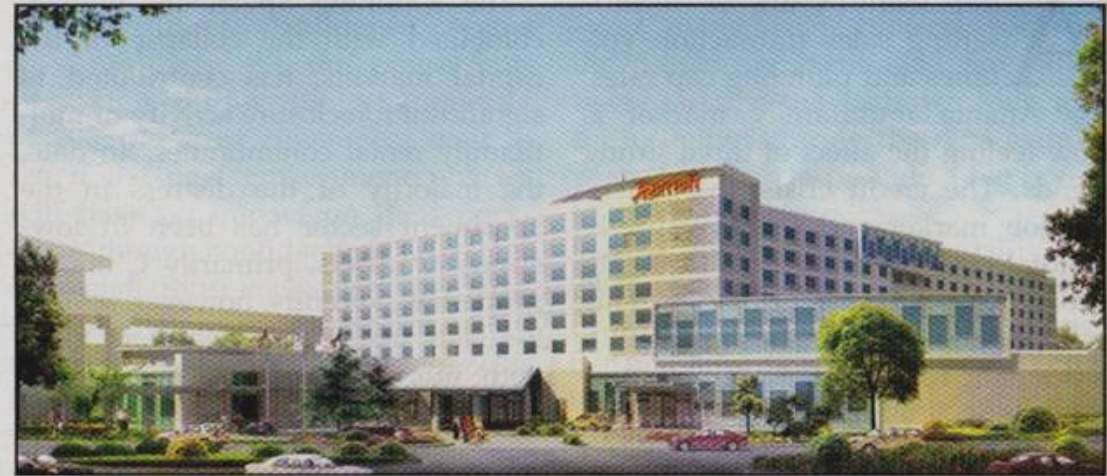
The $250 million Gateway Center development near the Hartsfield-Jackson Atlanta International Airport will house a Marriott and a Springhill Suites.
